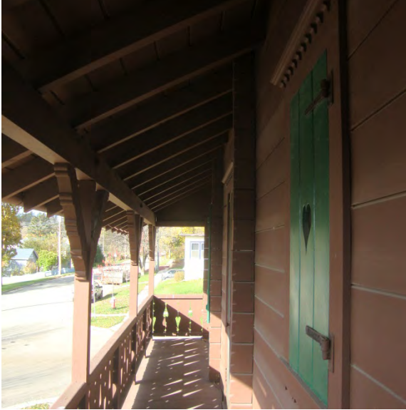
Image 1.10 View of the south balcony
